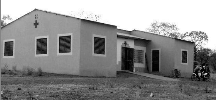
Figure 8: The new Sadiola district clinic
