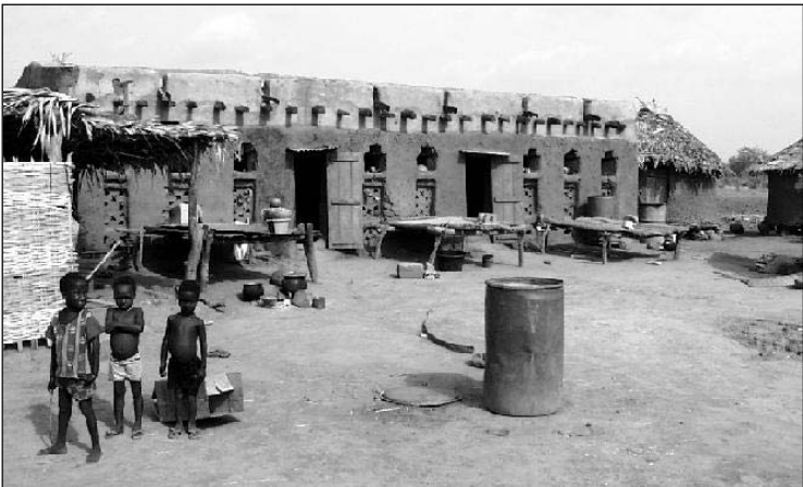
Figure 6: Example of a special design house in Niamboulama, features of which would need to be duplicated in the new village.
