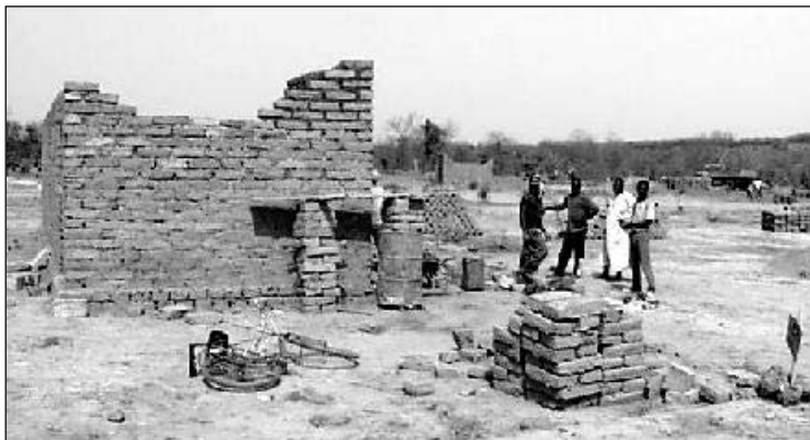
Figure 12: New Arrivals building replacement structures in the new Sadiola village. Bricks are made of mud and straw. Note the similarity of design to those provided to the Original Inhabitants - a departure from the traditional hut design.
