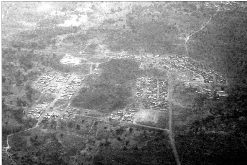
Figure 13: Aerial view of new Sadiola village – the New Arrivals are located to the west (right) of the central hill and the original inhabitants are on the eastern side (left). Note the modern layout adopted for the new village.
