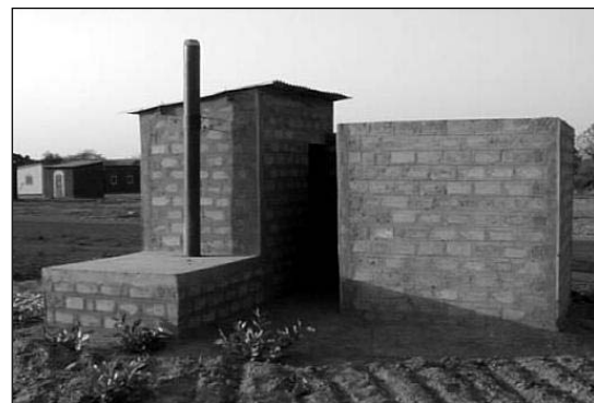
Figure 15: Kassatan 'no smell' toilet (& shower) (based on the SAfr pungalutho) has not been successfully introduced. Pit latrines are favoured.
